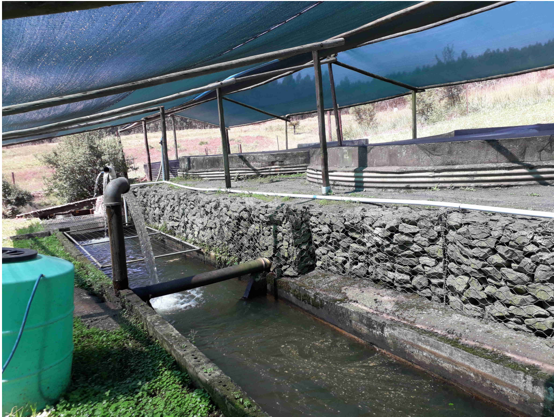
Figure 2.5: The Mbona raceway is used as an exit for the water after it has passed through the baths, tanks or ponds. It is also used to grow trophy and table fish for select customers.
